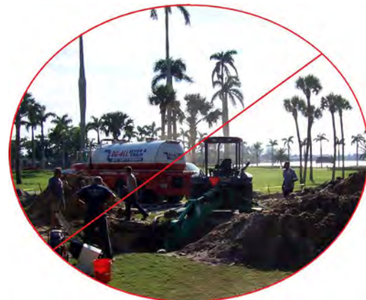
No Digging or Demolition
