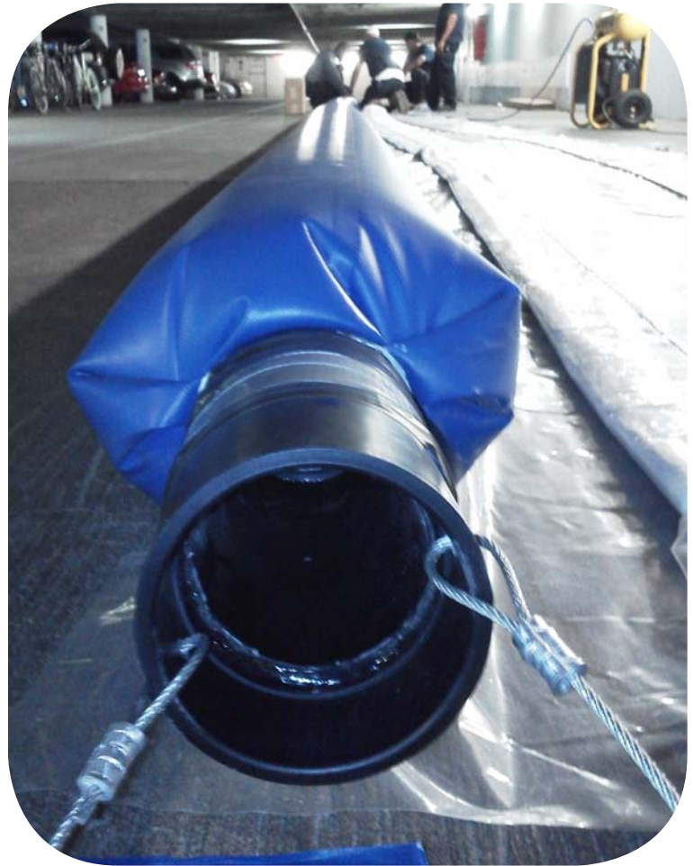
Nu Flow's unique flow-through system that acts as an internal bladder during the structural lining process, also keeps mains operational during our work.
